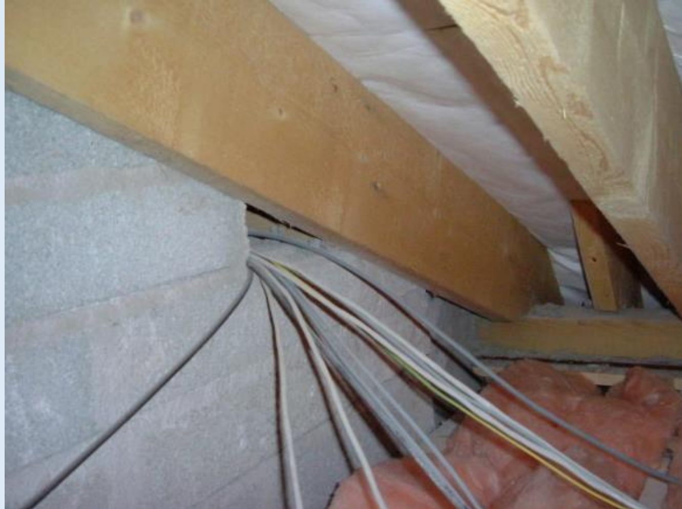
Compartment wall in 4 storey apartment building
