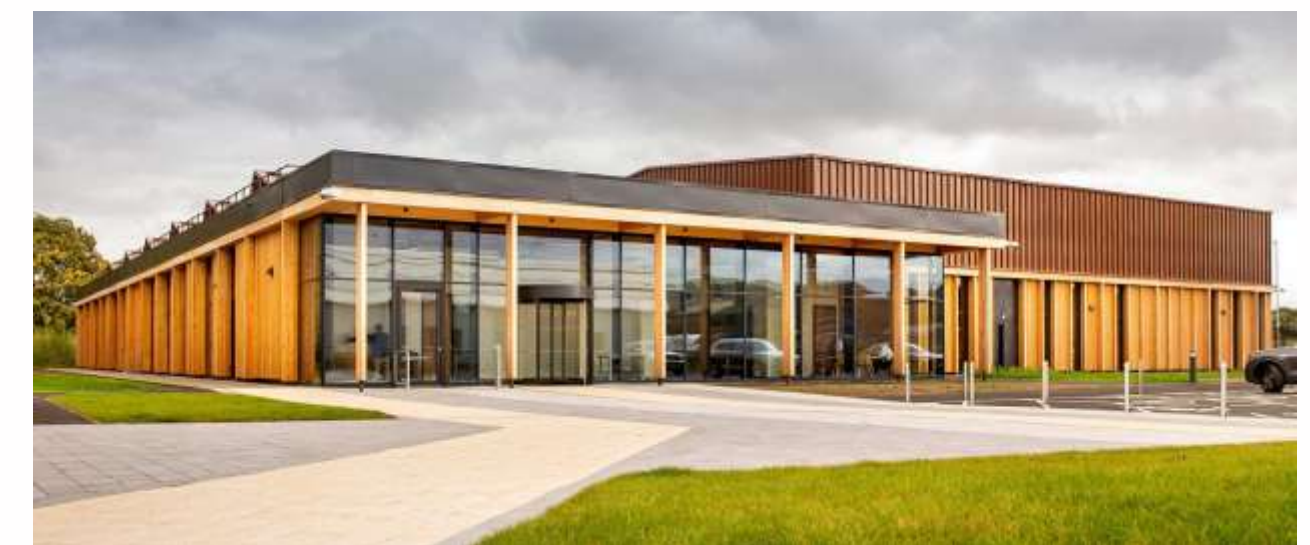
NMITE Living Lab, Transforming Timber UK
