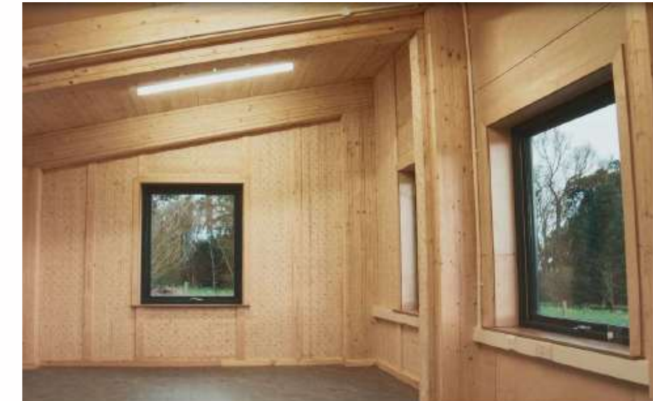
Dowel Laminated or Cross Laminated Timber (DLT or DCLT) e.g. floors, walls, roofs (see AFTB project on TERG website)
