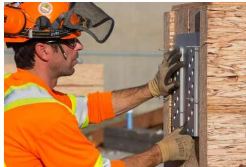
Parallel Strand Lumber (PSL) e.g. long span beams, columns
