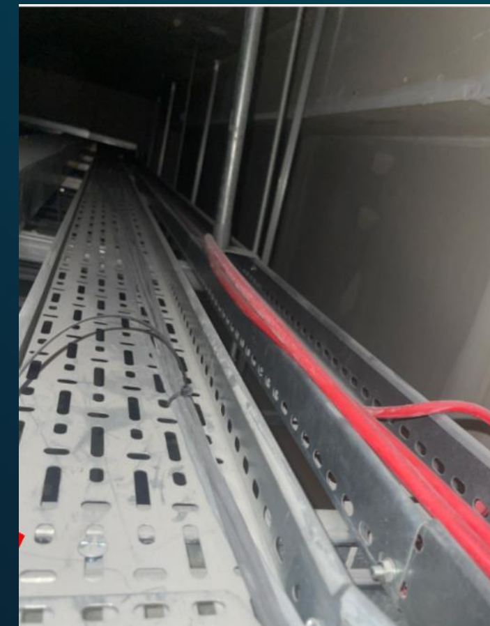
I.S. 10101 - Figure 44.RZ3 – Examples of maintenance of continuity of metallic system components to provide electromagnetic compatibility protection
