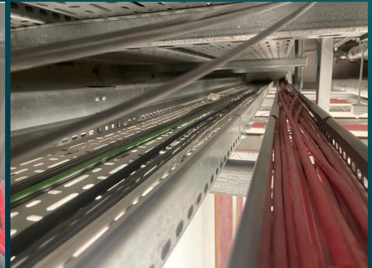
I.S. 10101 - Figure 44.RZ3 – Examples of maintenance of continuity of metallic system components to provide electromagnetic compatibility protection
