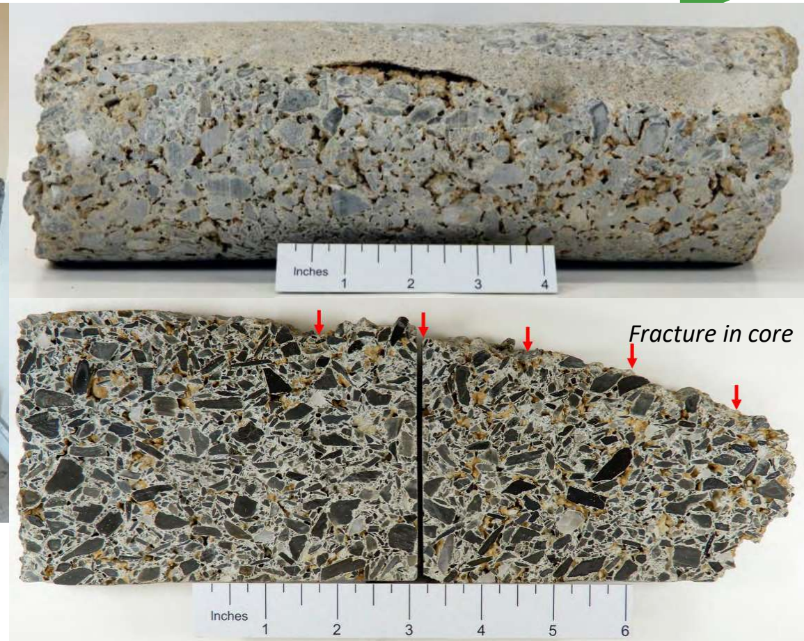
Images from Concrete Research & Testing Report No. R-190-1
